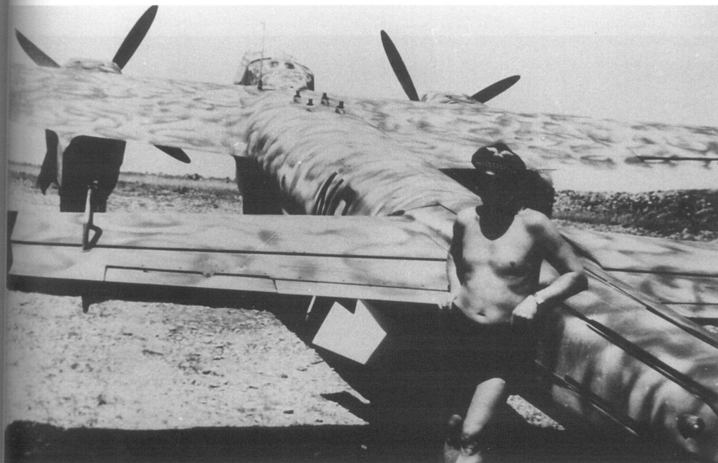
LEFT: This unusual configuration of six vertically mounted MG 151 cannon installation was first proposed by Stabs Ingenieur Poppendieck, an engineer at the E-Stelle at Werneuchen. Here it is seen installed in a Do 217 of the night fighter training Geschwader NJG 101. However, this conversion was not adopted in large numbers and night fighter pilots preferred the usual twin-cannon armament which became the standard configuration.
